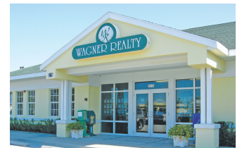
5215 SR 64 East Bradenton, Florida
